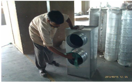
Cleaning Prior To Installation
