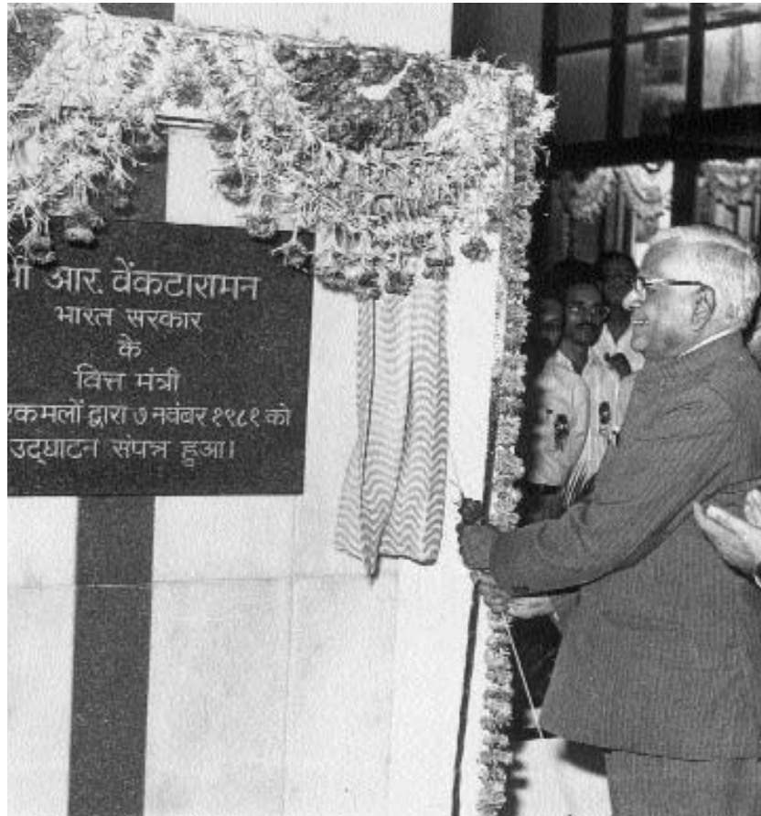
31 Finance Minister R. Venkataraman inaugurating the new Central Office Building, Bombay
