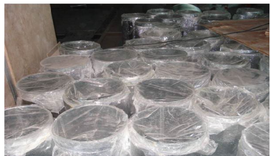
Ducts Stored with Properly
