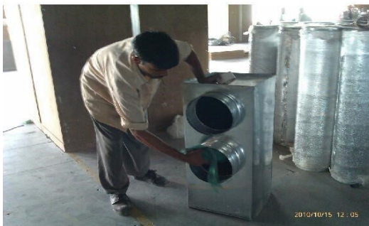
Cleaning Prior To Installation
