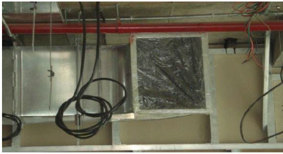
Ducts Wrapped With Plastic to Avoid Dust Wrapped
