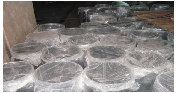
Ducts Stored with Properly with Plastic
