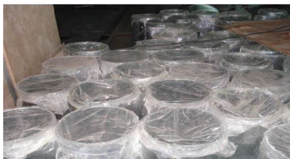
Ducts Stored with Properly Wrapped with Plastic
