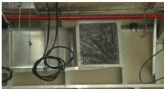
Ducts Wrapped With Plastic To Avoid Dust
