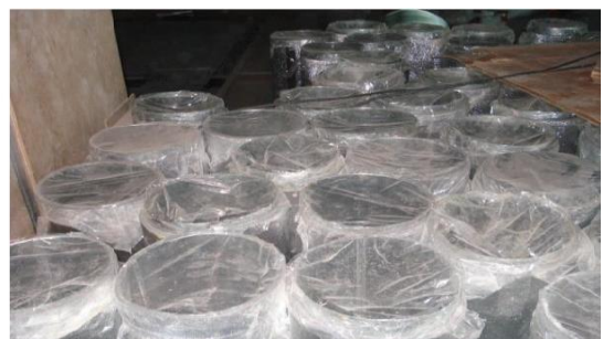
Ducts Stored with Properly Wrapped with Plastic
