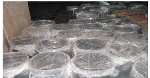
Ducts Stored with Properly Wrapped with Plastic
