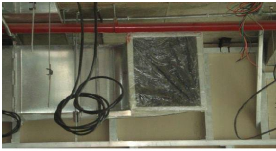
Ducts Wrapped With Plastic to Avoid Dust
